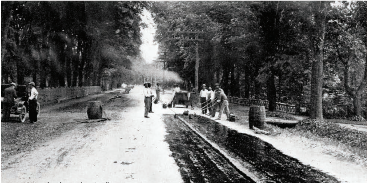
Preparing road surfaces with tar in Albany County. Right: Adirondack road construction map
